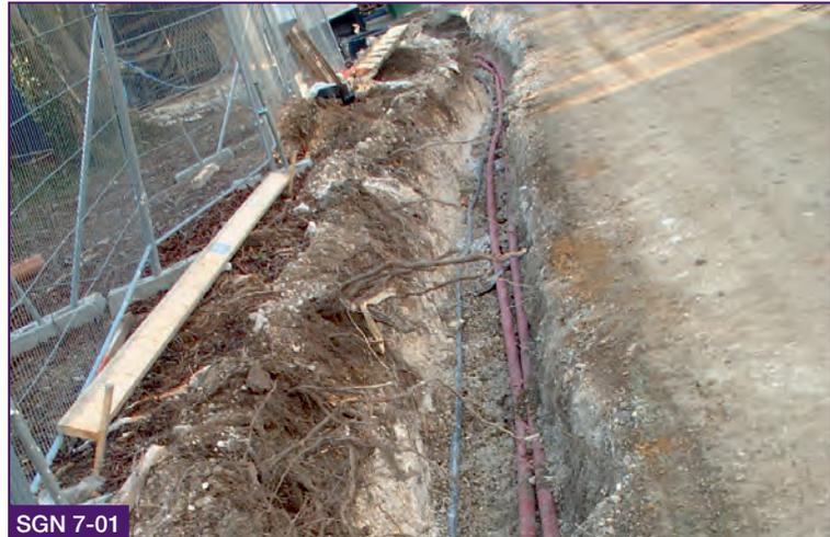
All excavation in RPAs should be with hand-held tools. Where possible, there will be a preference to use air tools because they are very effective at exposing roots and services with minimal damage.
