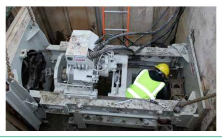
SGN 11-03 Thrust boring is the preferred option for installing service routes through the RPAs of retained trees.
