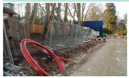
SGN 11-01 Conventional installation of services digging a trench with a machine is not permitted in RPAs.
