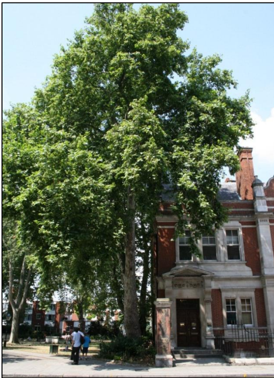
Trees can cause significant structural damage. The expertise of consulting arborists is needed to find sustainable solutions that allow trees and structures to coexist.
