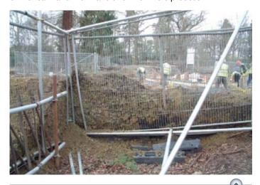
Braced fencing is important because it is difficult to imagine the pressures that have to be withstood when writing the specification in the comfort of the office!
