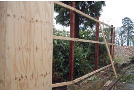
High specification ply fencing fixed to a robust wooden framework is effective at protecting trees
