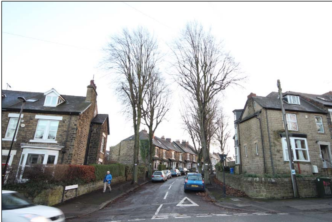
Many of the trees in Ladysmith Avenue are under threat of felling because of surfacing damage.
