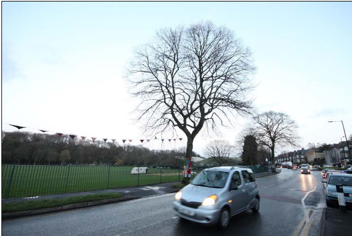
Two mature trees on Rustlings Road scheduled for felling due to highway damage (see Photo 2 for a close up).
