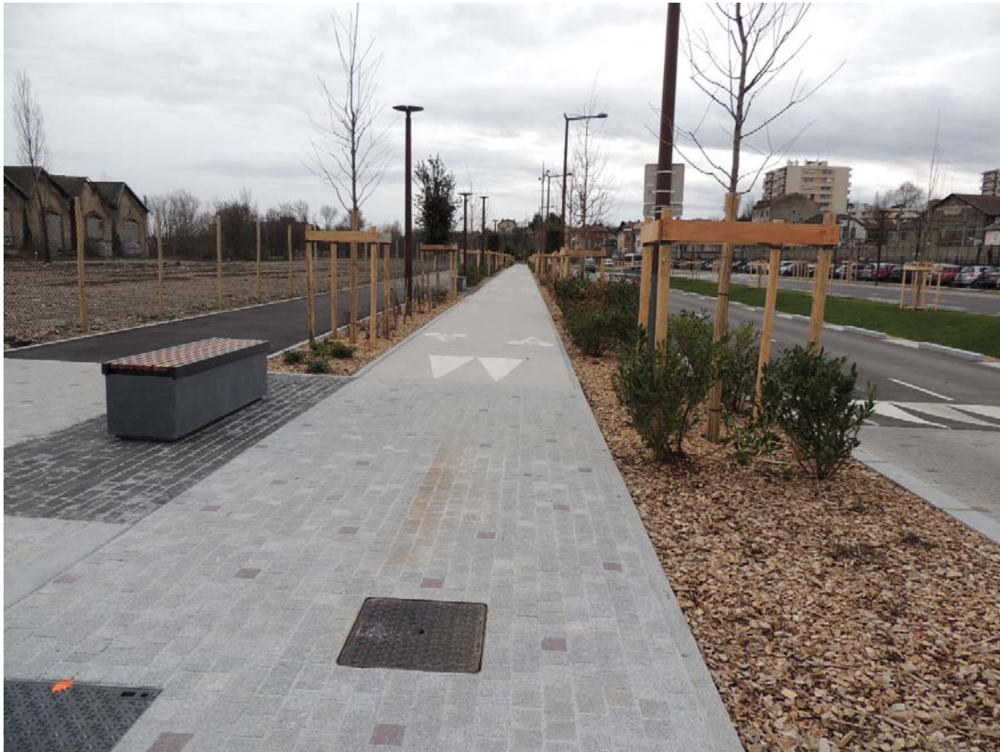
Highway futures here today in Lyon, France; planned integration of pedestrians, cyclists, vehicles and trees.
